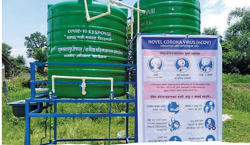
« Contactless handwashing facility with the provision of drinking water installed in Bardiya.
