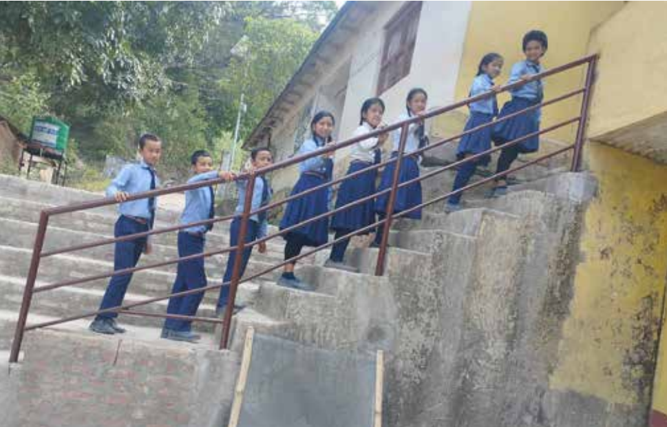
Establishment of Fencing for maintaining the school safety standards
