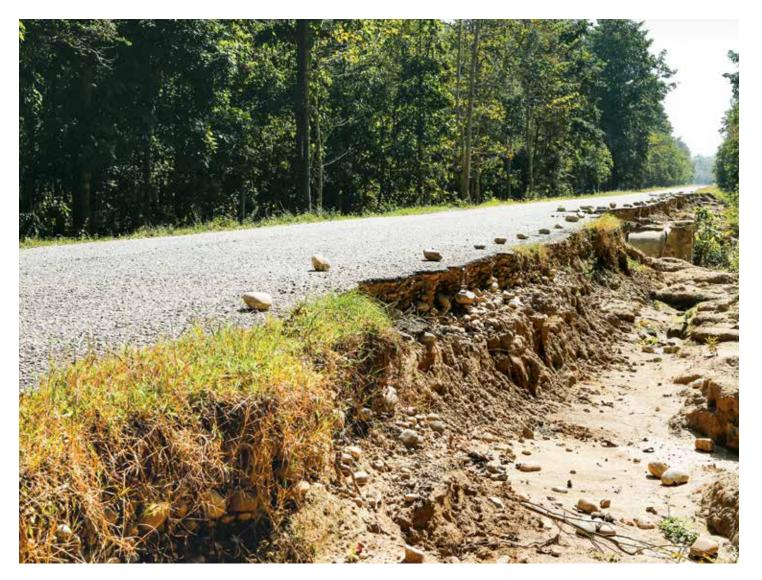
Mahendra Highway (East West Highway) damaged by floods and in a very poor stage that needs immediate maintenance
