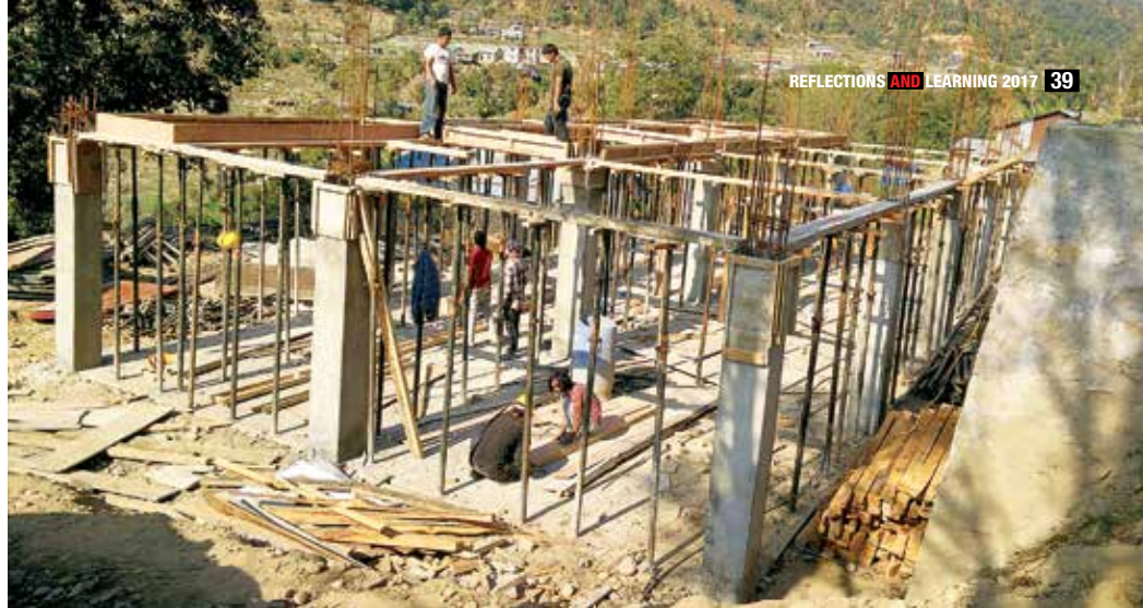
School construction of Sindhupalchowk in progress.
