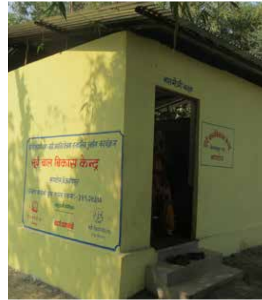
▲ Construction of an Early Childhood Development Centre in a flood affected area of Morang.
